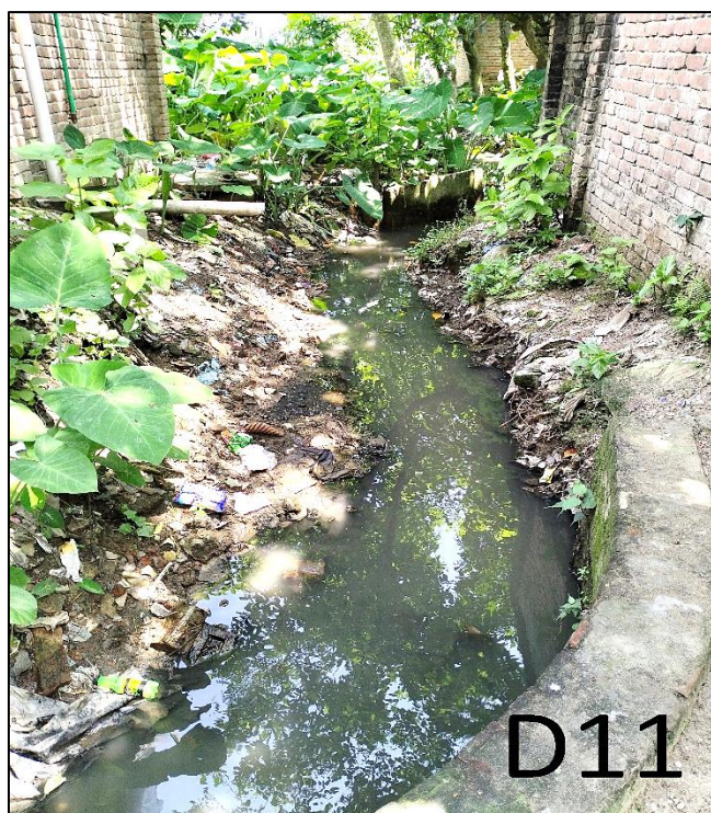
BHER-D-11:. Construction of RCC Drain from infront of Paurashava to existing Hazipara Lake Drain, Ch.0.00 - 895.00m, Total Length = 895.00m at Nawdapara & Bamonpara Ward No.03 & 09, under Bheramara Paurashava, Kushtia.
